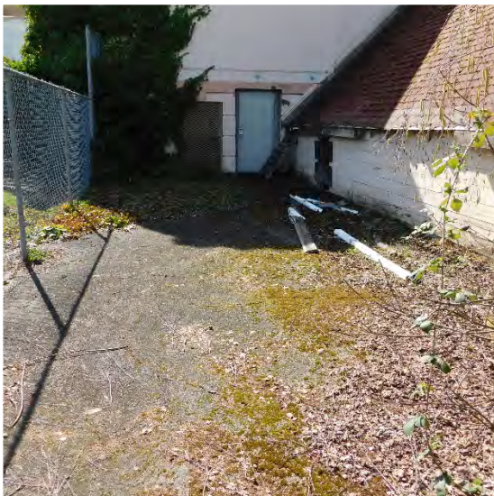
Asphalt pour to building with no protection from building
