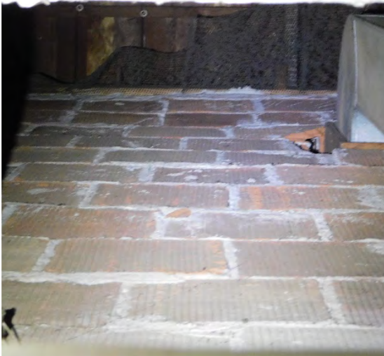
Exposed masonry walls to roof structure
