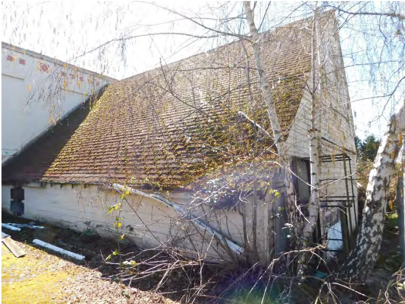
Figure 2 East Elevation of North Building
