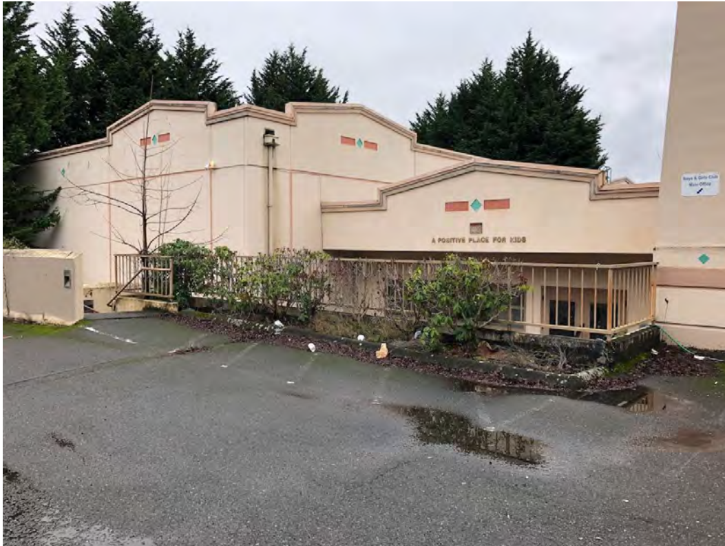
Looking southwest at the east side of the 1990 gym addition.
