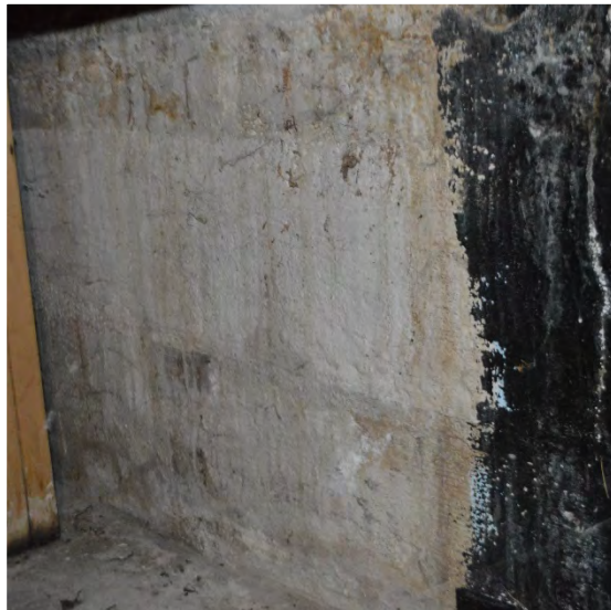
Exposed concrete walls with no finish
