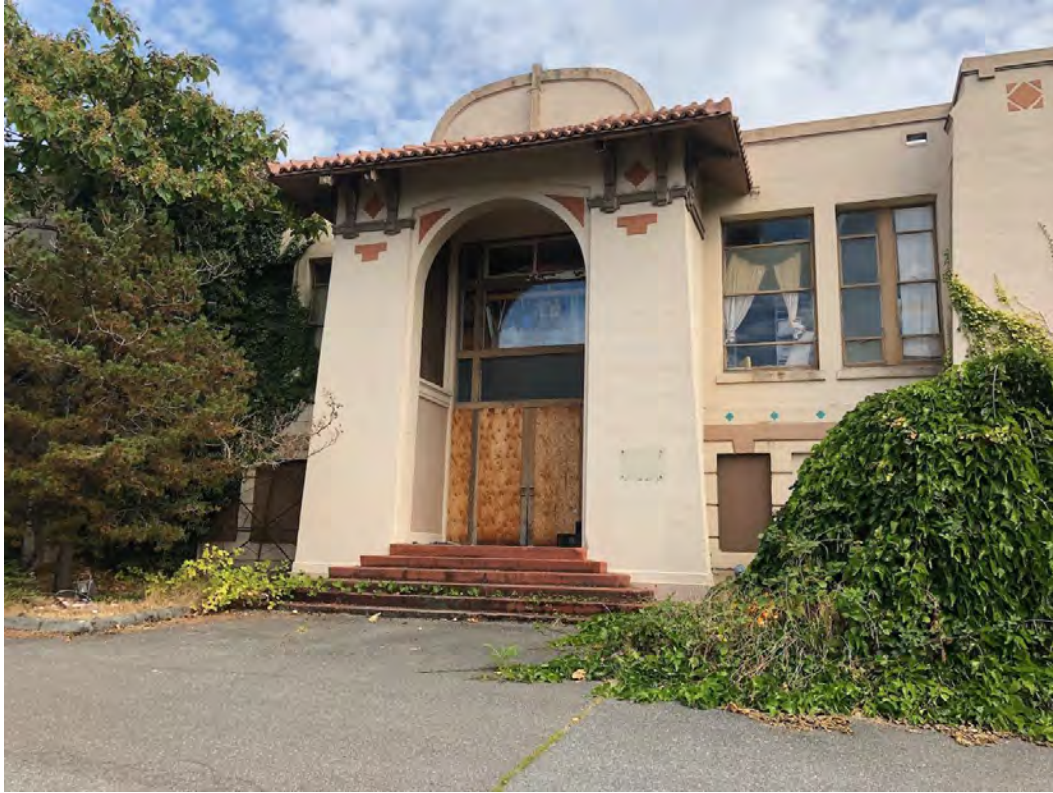
Former main entry, west façade. (September 2019)
