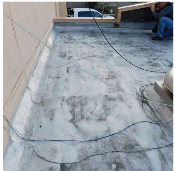
Roof flat with slight slope with built-up roofing.
