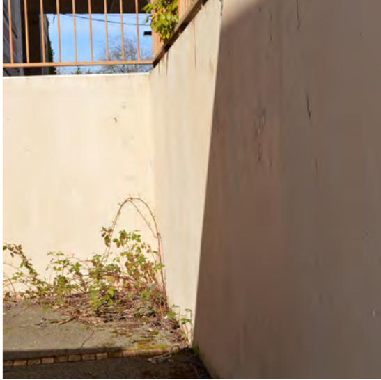
Guardrail rusted, wall punctured
