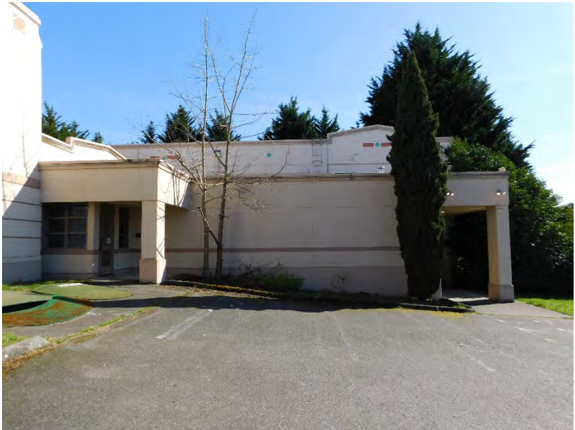
Figure 2 Southwest Elevation at South Building - Gymnasium
