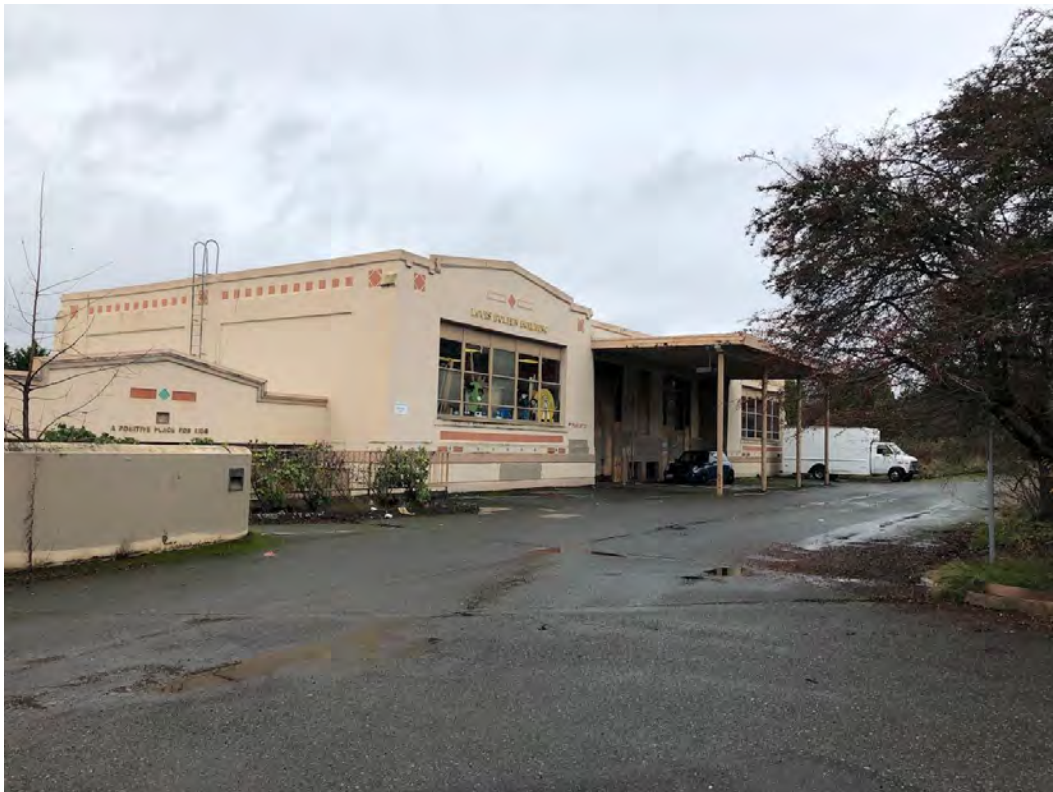
Looking northwest from the east parking lot, toward the east façade.
