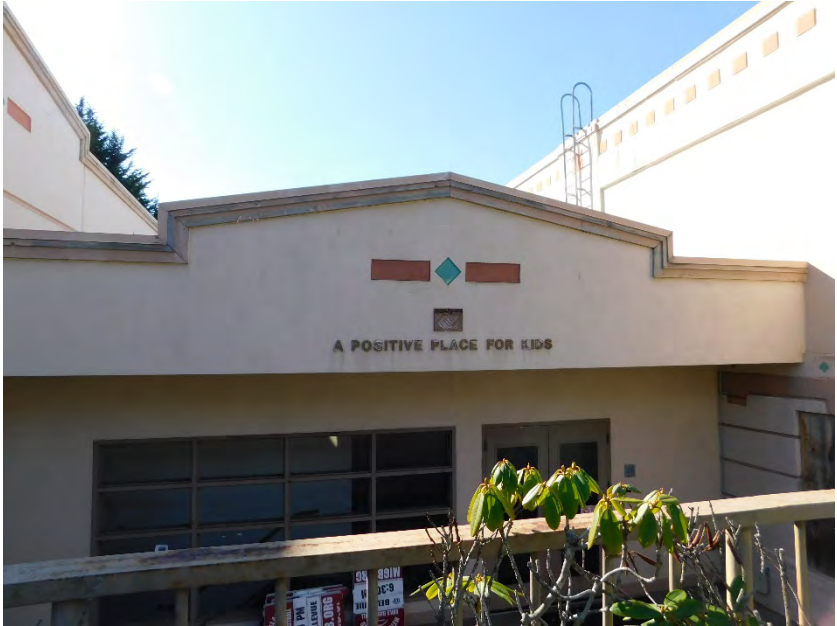
Figure 1 East Elevation at North Building - Gymnasium
