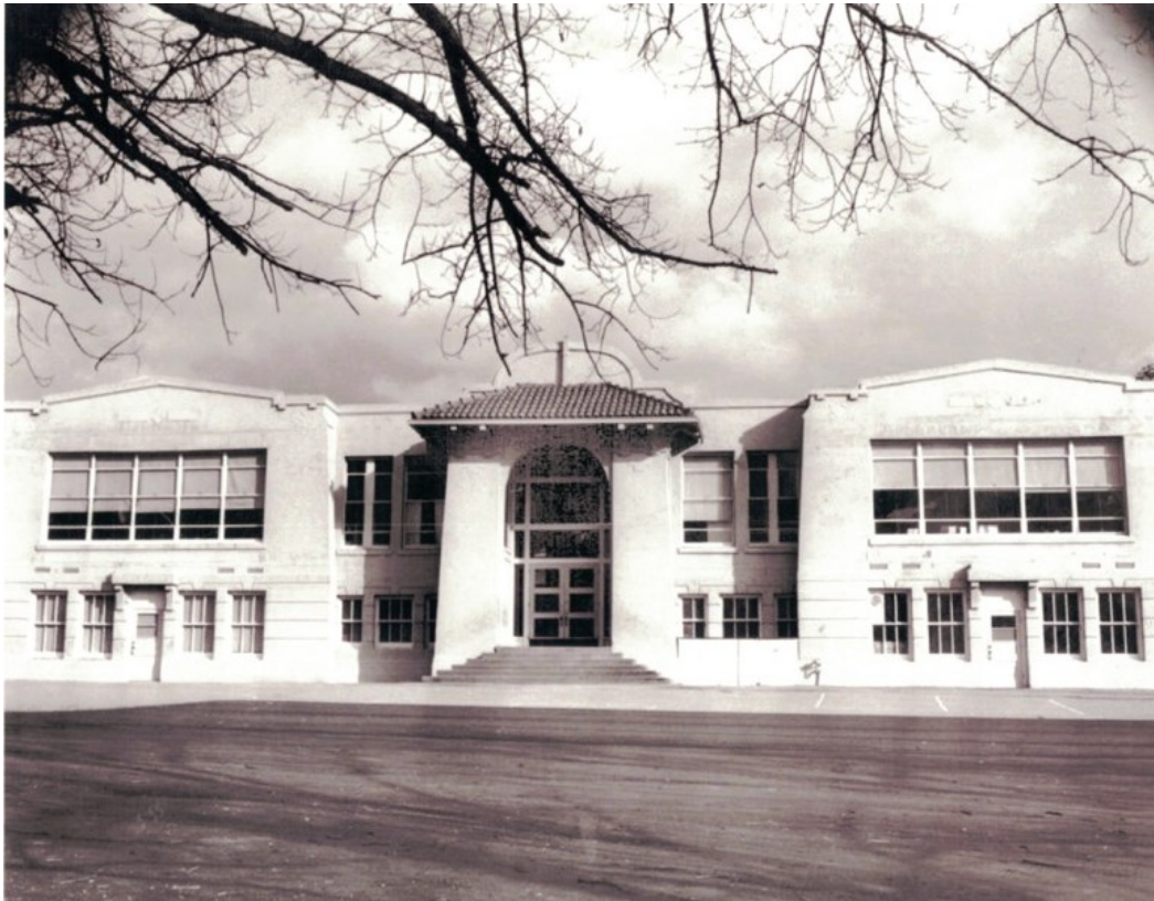
Undated, pre 1965 view of the primary west facade
