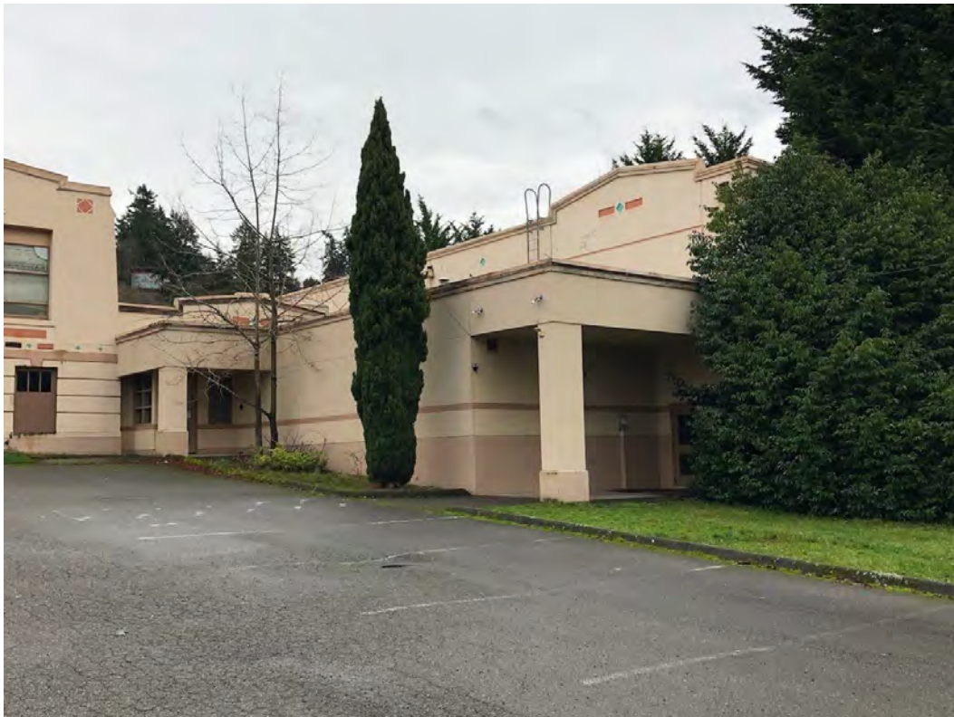
Looking southeast from the west parking lot, toward the 1990 gym addition.
