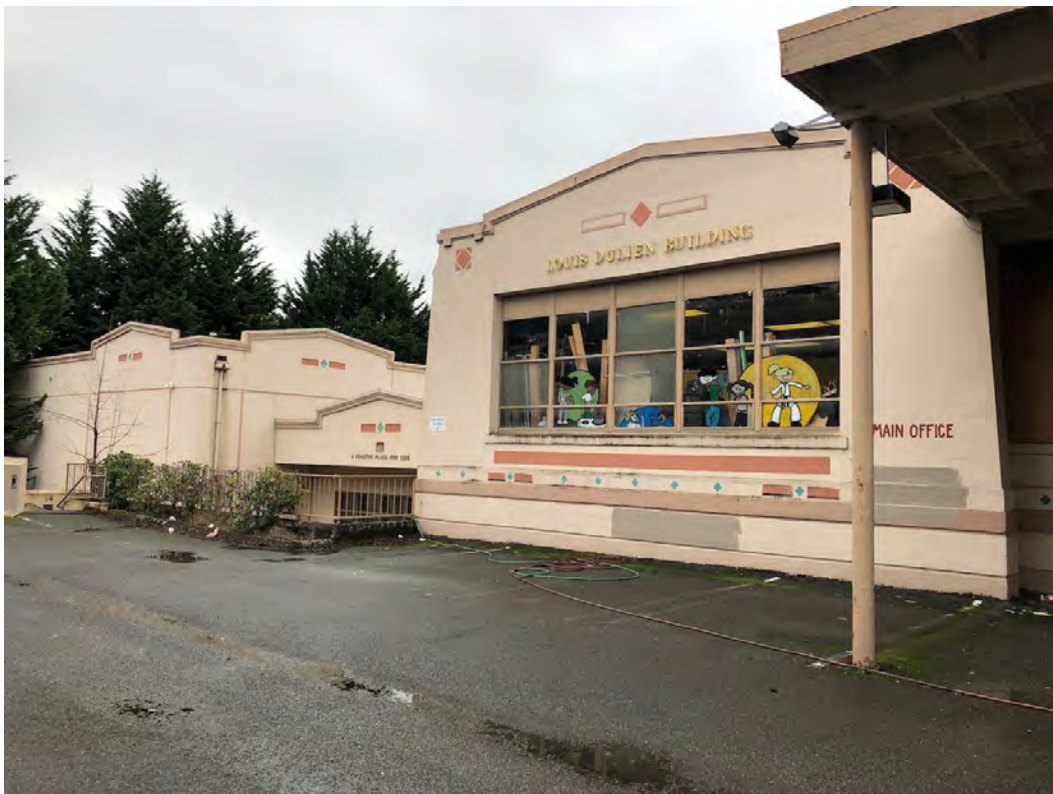
Looking southwest at south end of east façade and 1990 gym addition beyond.
