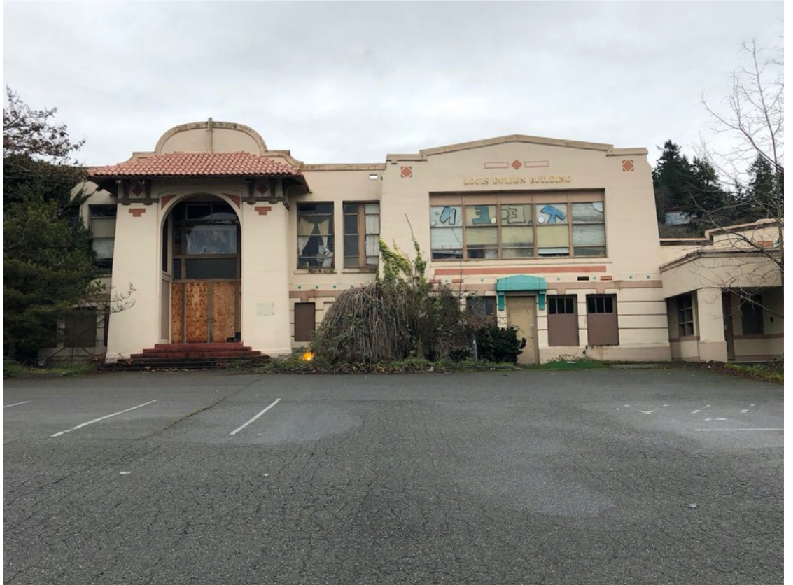
View looking east toward southern portion of the west façade, with 1990 gym addition partially visible at the right edge of photo
