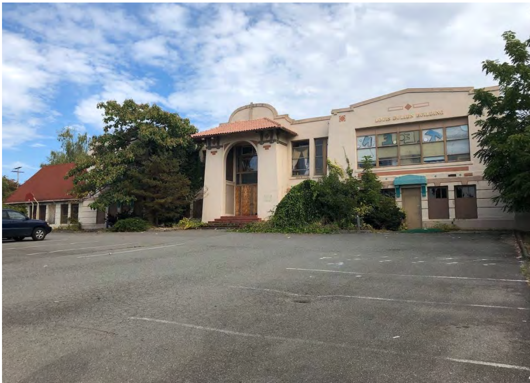
Looking northeast toward the west façade, from the west parking lot. (September 2019)
