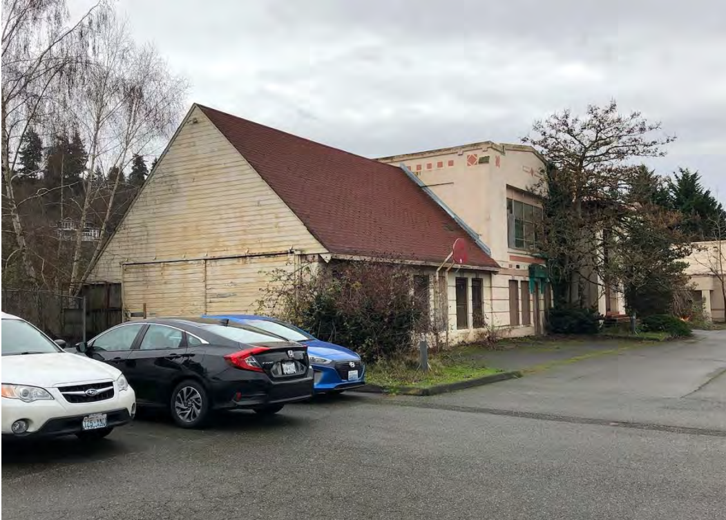
Looking southeast from the north end of the building, with the playshed addition in the foreground.
