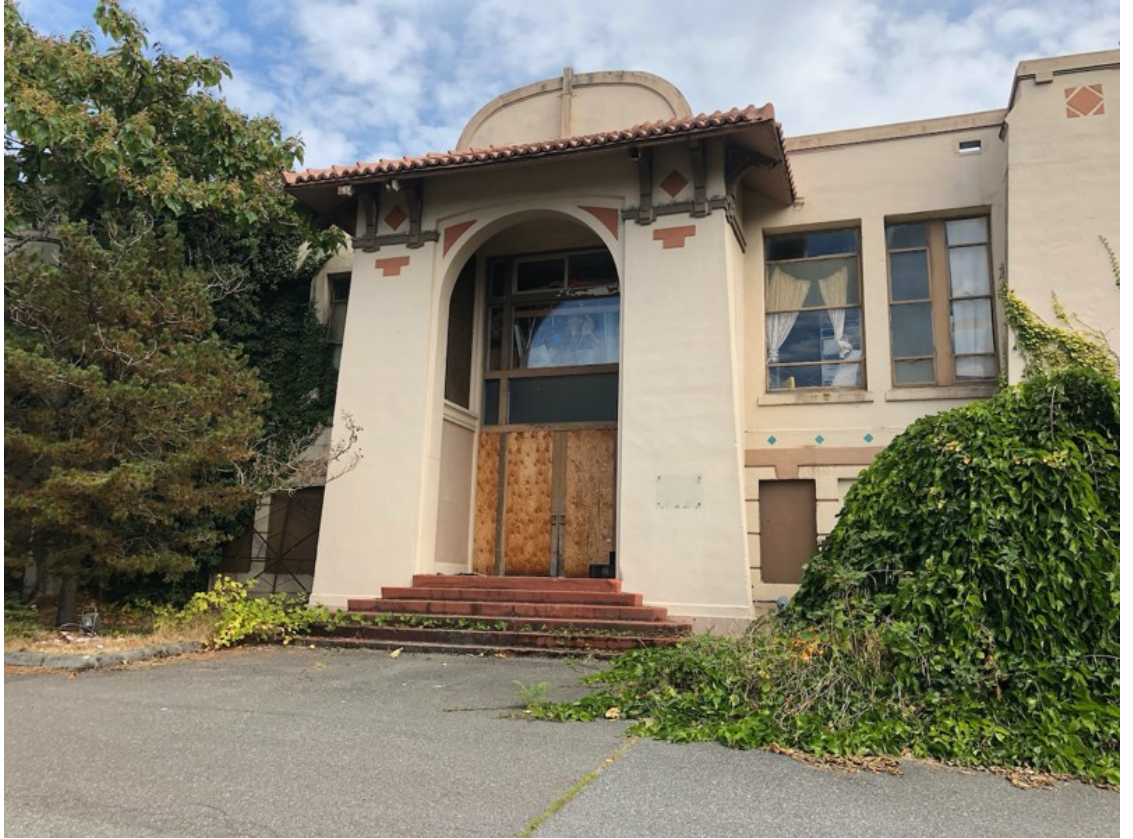
Former main entry, west façade
