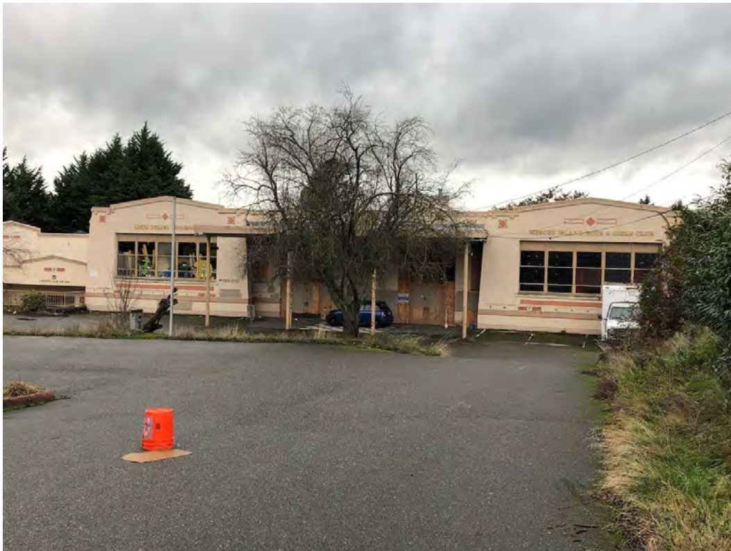
Looking west toward the east façade, from the driveway off West Mercer Way.
