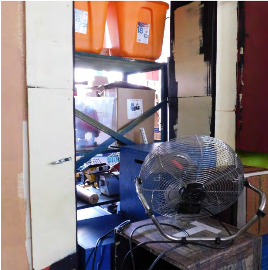
Access entries added between rooms with no doors.
